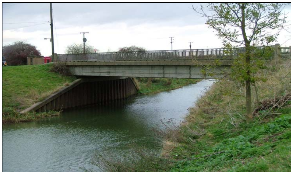
Photograph 5.1 - Tetney Lock Main Bridge
