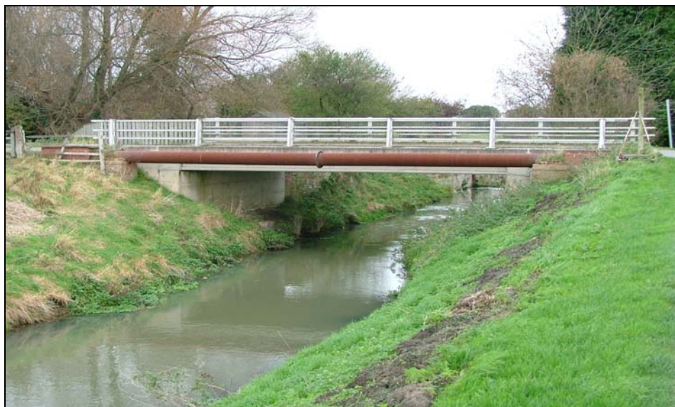
Photograph 5.11 - Alvingham Lock Bridge and Pipebridge (water main)
