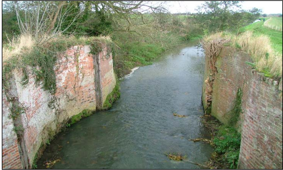
Photograph 4.5 - Ticklepenny Lock – Note gates have been removed
