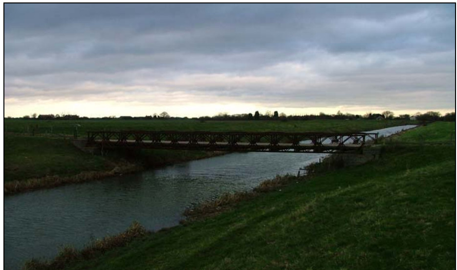
Photograph 5.2 - Riverside Farm Bailey Bridge
