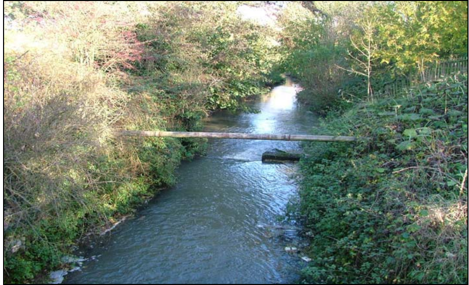
Photograph 8.2 - Water main downstream of Keddington Church Lock
