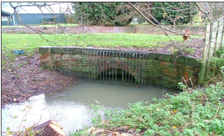
Photograph 7.2 - Alvingham Upper Syphon and Mill Stream (Upstream side)
