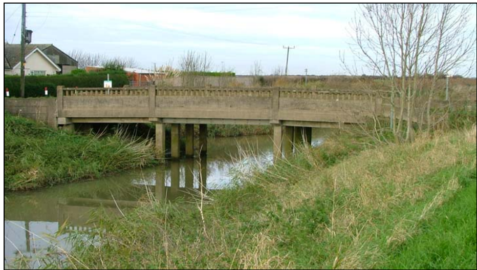
Photograph 5.7 - Austen Fen Bridge
