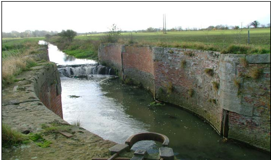
Photograph 4.4 - Willows Lock – Note gates have been removed
