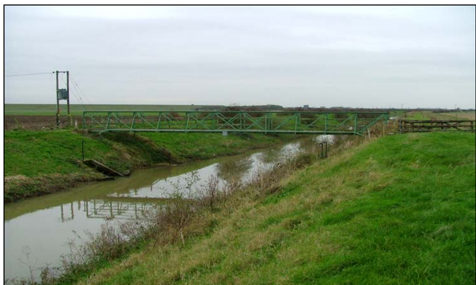
Photograph 5.6 - Biergate Foot Bridge and outfalls from LMDB Biergate Pumping Station
