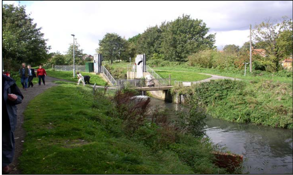
Photograph 5.15 - Environment Agency Louth Tilting Weir and foot bridge on site of Old Top Lock
