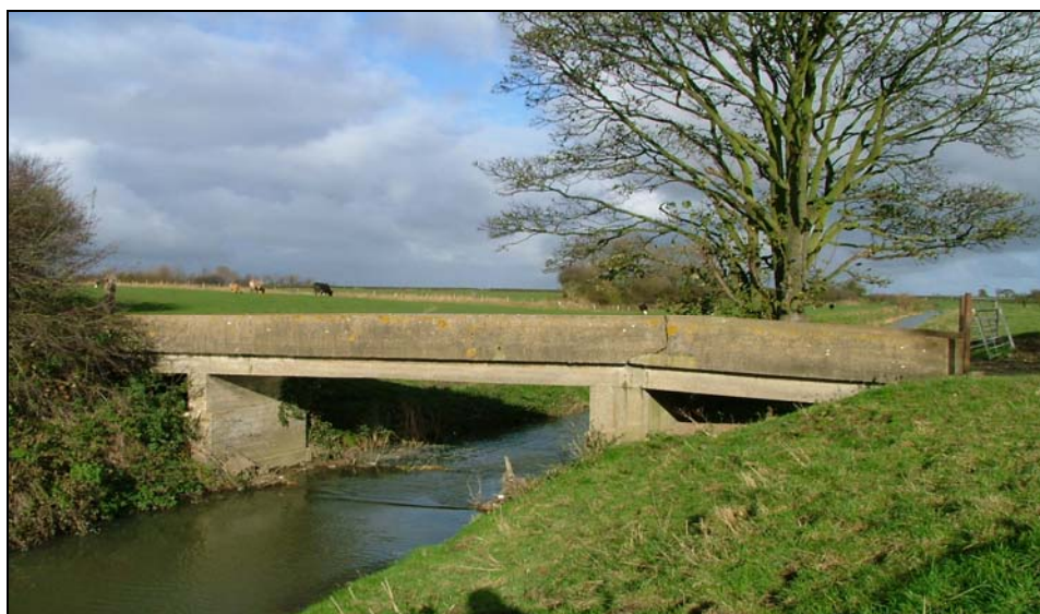
Photograph 5.12 - River Farm Access Bridge
