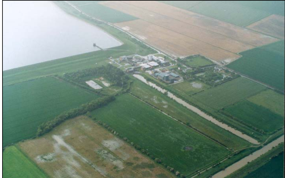
Photograph 2.4 - Covenham Reservoir and intake channel from the Louth Canal
