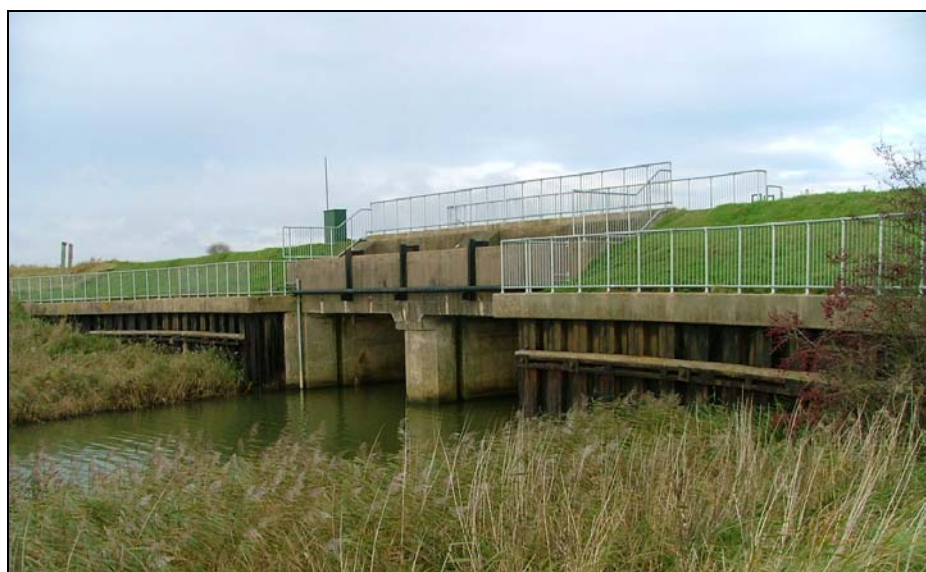
Photograph 2.3 - Tidal outfall to Tetney Haven
