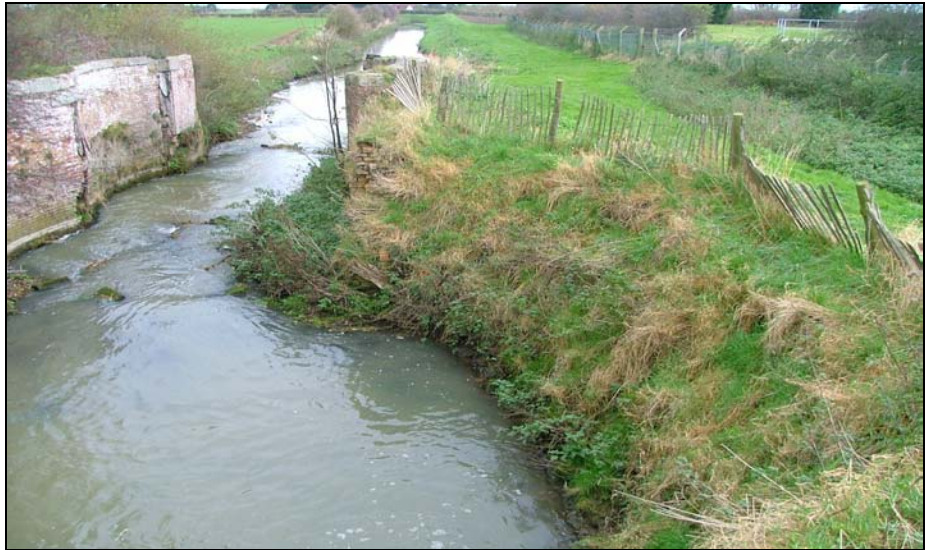
Photograph 4.3 - Salterfen Lock – Note gates have been removed
