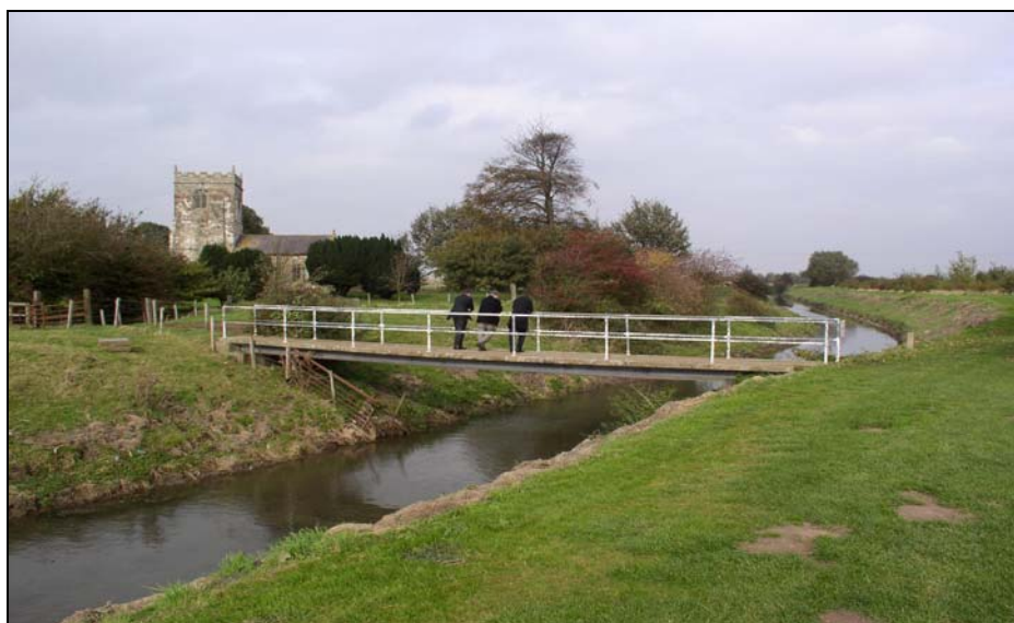
Photograph 5.10 - Alvingham Canal Church Foot Bridge viewed from upstream
