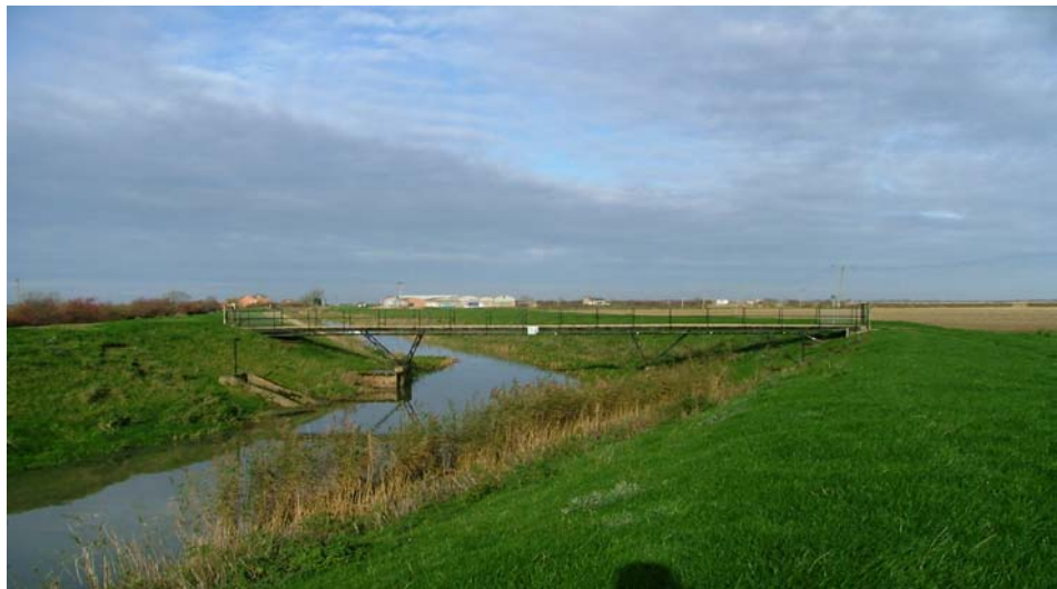
Photograph 5.8 - Austen Fen Foot Bridge and outfalls from LMDB Austen Fen Pumping Station
