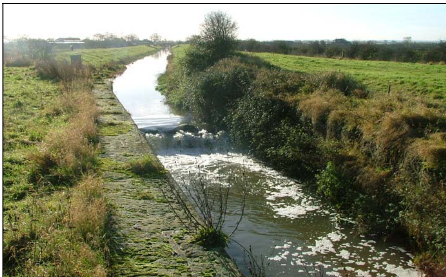
Photograph 4.1 - Outfen Lock – Note gates have been removed
