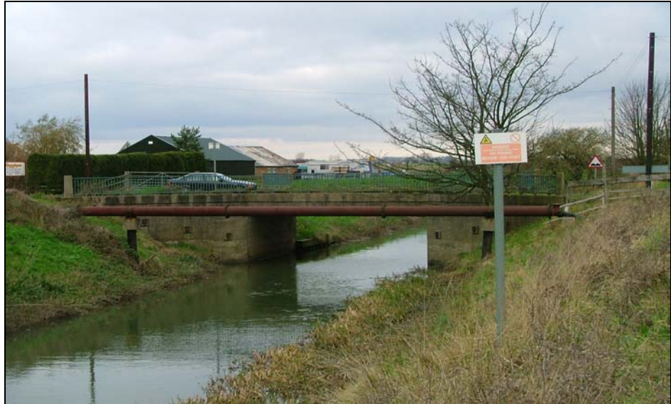
Photograph 5.5 - Fire Beacon Bridge and Pipebridge (water main)
