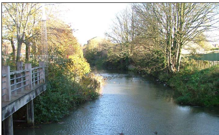
Photograph 2.2 - Louth Canal - Riverhead
