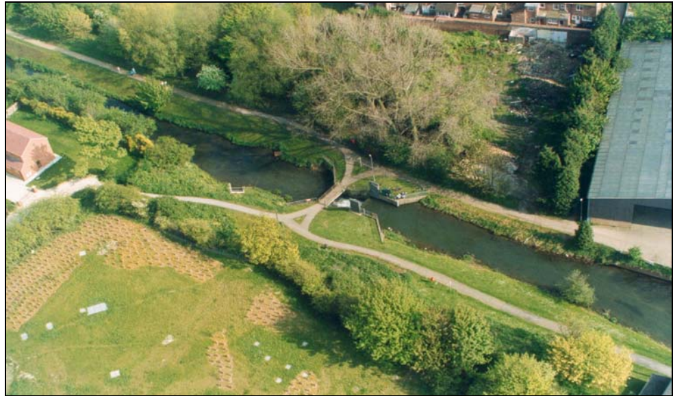
Photograph 4.7 - Environment Agency Louth Tilting Weir on site of old Top Lock
