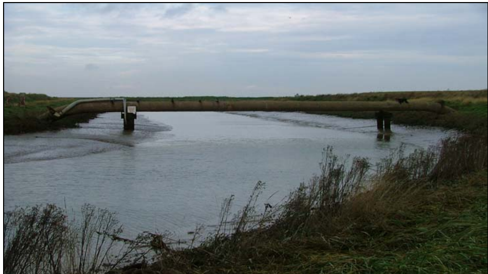
Photograph 8.4 - Oil Transfer Pipeline across Tetney Haven
