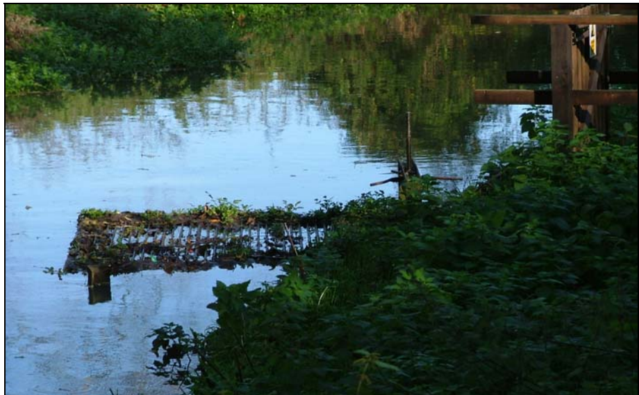
Photograph 7.1 - Sluice for compensation flow to River Lud upstream Keddington Church Lock
