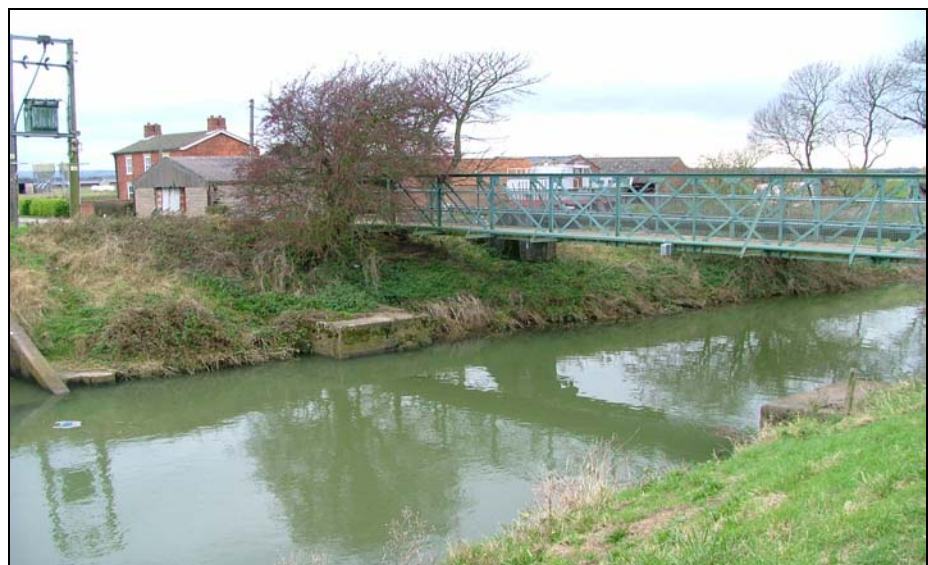
Photograph 5.4 - Fulstow footbridge and outfalls from LMDB Fulstow Pumping Station
