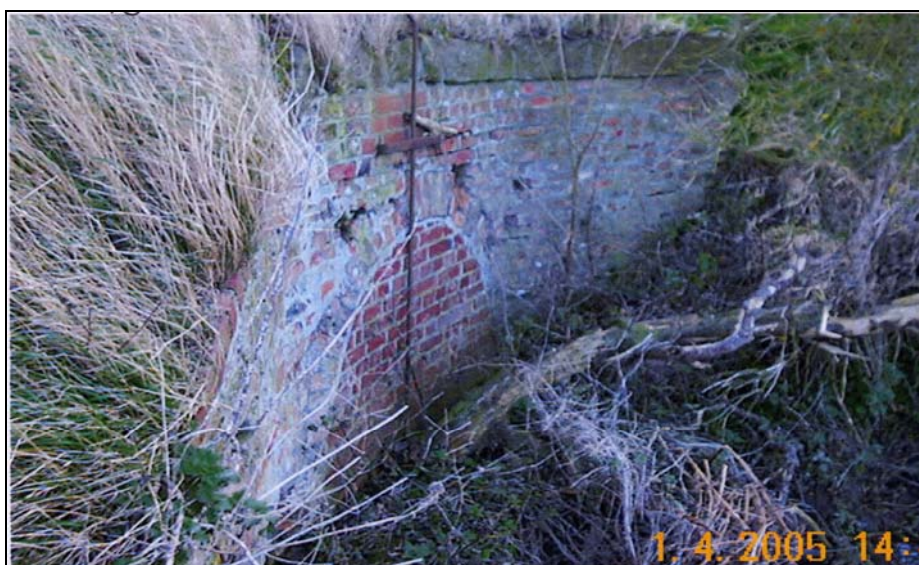
Photograph 7.4 - Abandoned and Bricked up Alvingham Lower Syphon (Upstream side)
