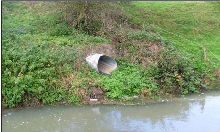
Photograph 8.6 - LMDB South Drain Outfall, downstream of Alvingham Lock
