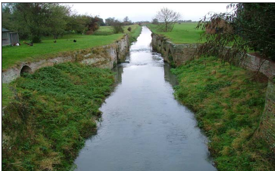
Photograph 4.2 - Alvingham Lock – Note gates have been removed
