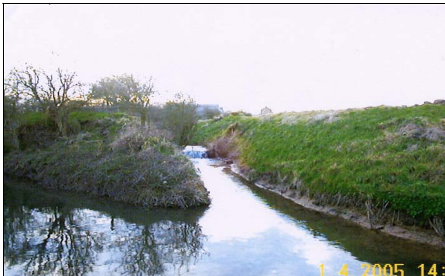
Photograph 7.3 - Lindsey Marsh Drainage Board Westfield Drain Weir
