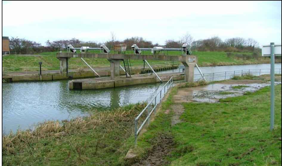
Photograph 7.6 - Anglian Water Tilting Weir downstream of Tetney Lock
